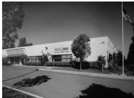
Current NECA/IBEW Electrical Training Center
